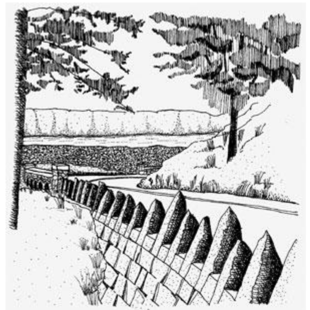
This image of a retaining wall with guard rocks shows ashlar patterns. Image provided by Oregon Historical Society (Library of Congress, Prints & Photographs Division, HAER ORE, 26-TROUT.V1- (sheet 12 of 27))
