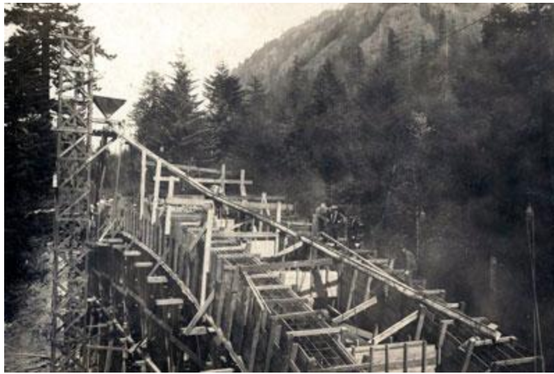
Workers prepare to pour concrete into forms with rebar during the construction of the Moffett Creek Bridge in 1915. (Oregon Department of Transportation)
