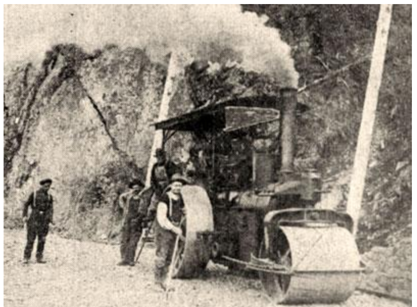
A steam roller compresses crushed rock before paving west of Hood River in 1920. (Portland Sunday Oregonian, March 28, 1920, Section 6, Page 1)
