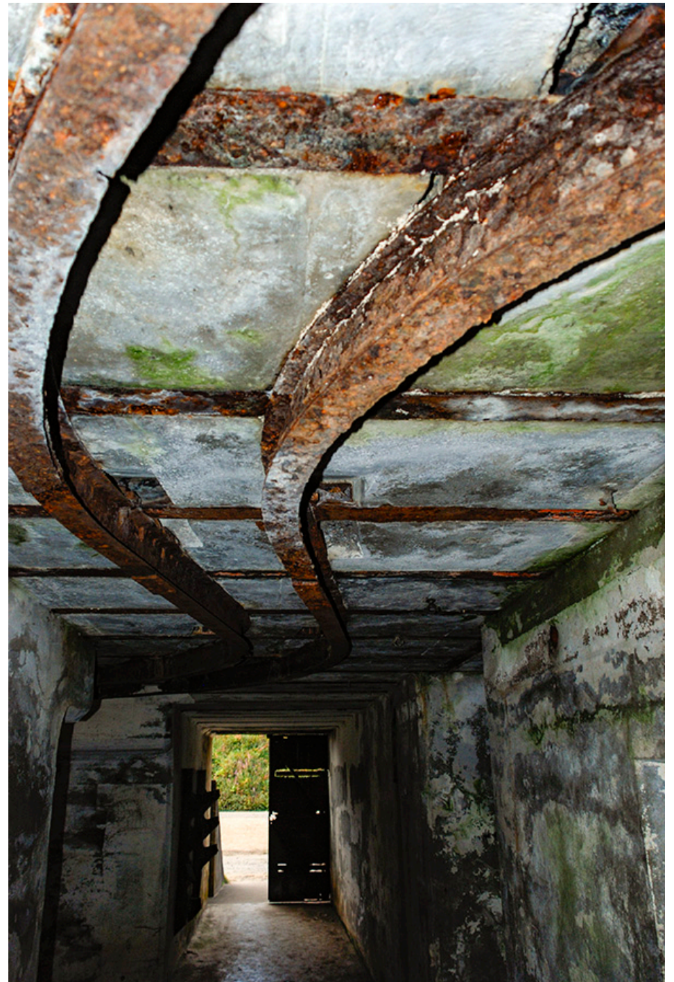
Overhead rails helped transport heavy munitions through the fortified West Battery at Fort Stevens. (Oregon State Archives, 2010)
