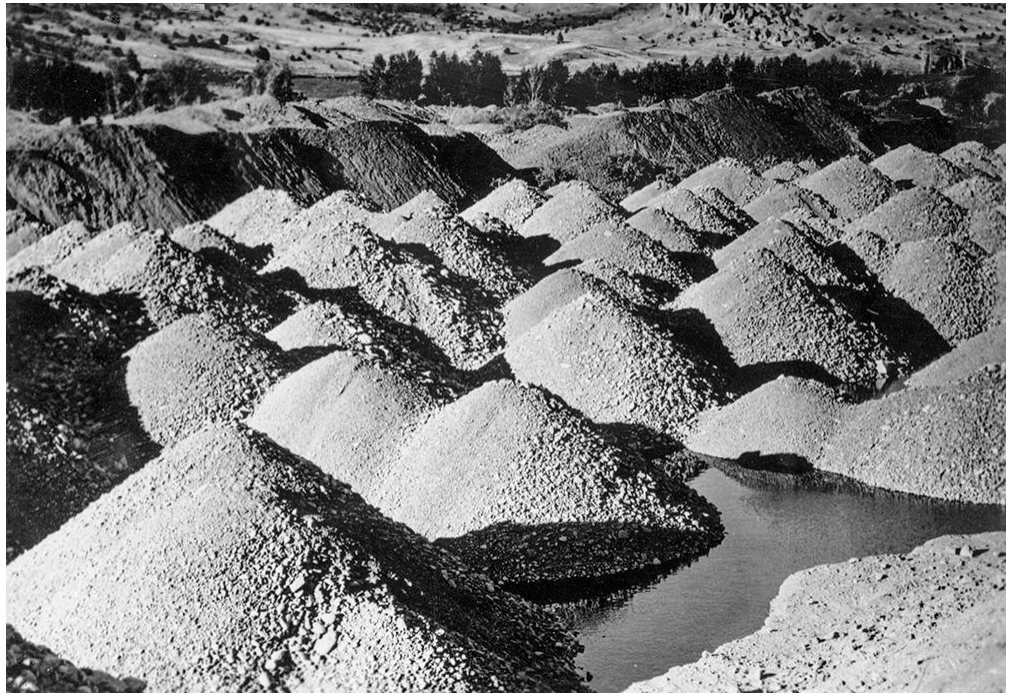
This 1938 photo shows a typical waste area, or tailings, from hydraulic dredge mining operations in Grant County. (Courtesy of Oregon Historical Society)
