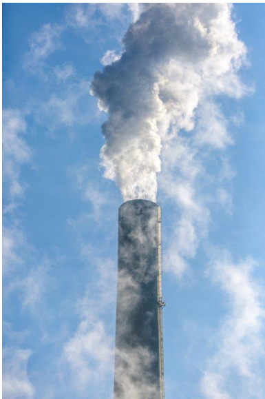
Steam from a smoke stack at an electric power plant.
