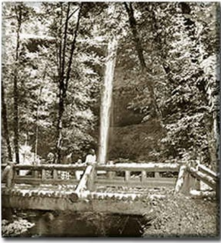
Silver Creek Falls Bridge (Highway Division photo #2569)
