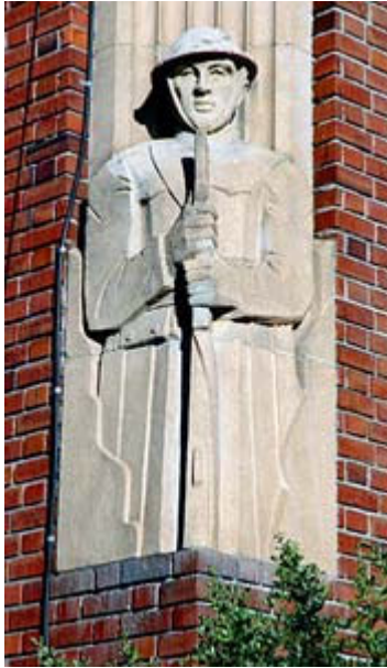
World War I era soldiers stand guard over the corners of the 1935 Art Deco style armory in Klamath Falls. The building houses the Klamath County Museum.
