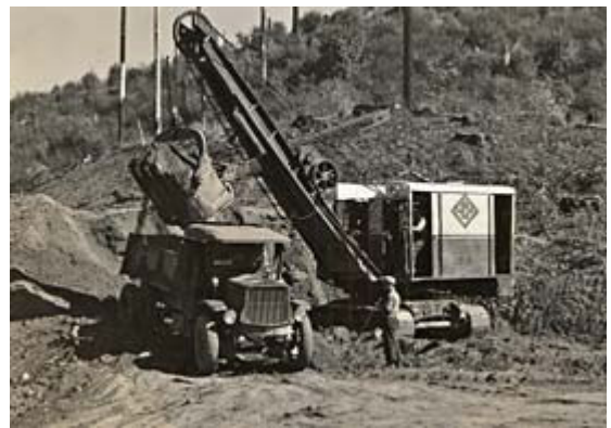
WPA workers construct the Wilson River Highway through the Coast Range in 1937.
