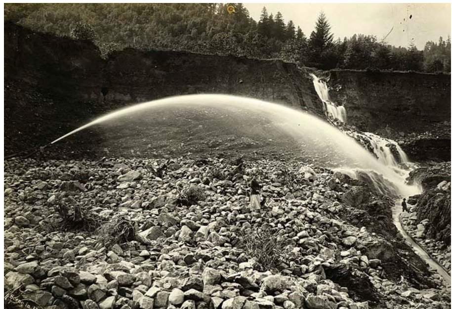
A water cannon blasts rocks from hillsides for gold mining. (Image courtesy Online Archive of California)
